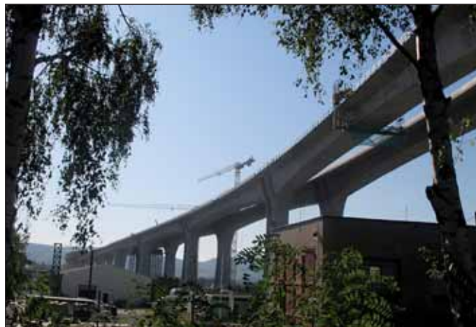
Obr. 2 Most u Radošína (st. 514) Fig. 2 The bridge near Radošín (lot 514)
