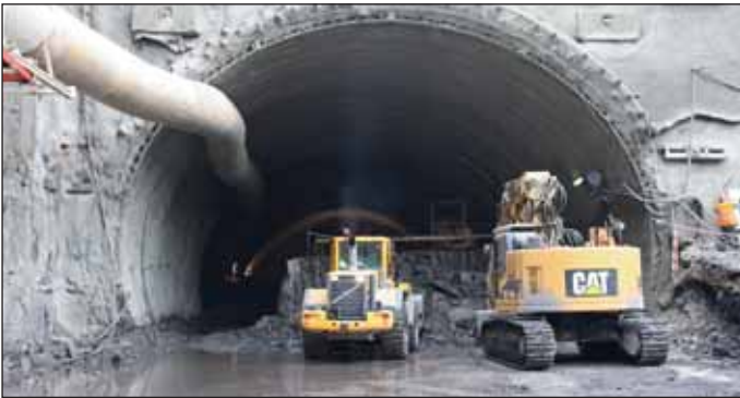
Obr. 3 Ražený tunel Brusnice Fig. 3 The Brusnice mined tunnel
